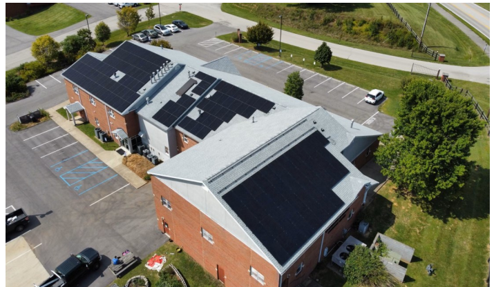
Photo: 68 KW-DC solar array on roof of Franklin County Cooperative Extension Office.
